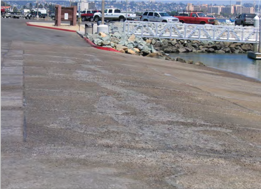
Worn Concrete Ramp
