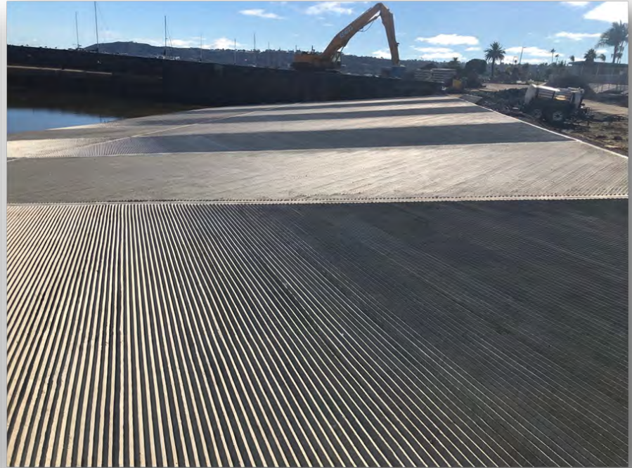
New V-grooved Concrete Boat Ramp
